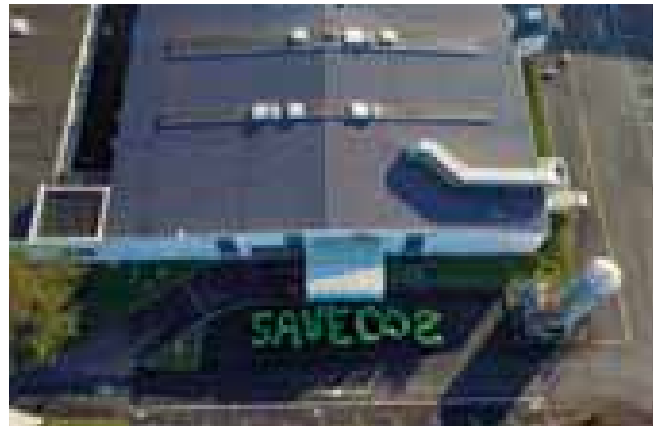
Schneider Electric’s Bourguebus site, France
